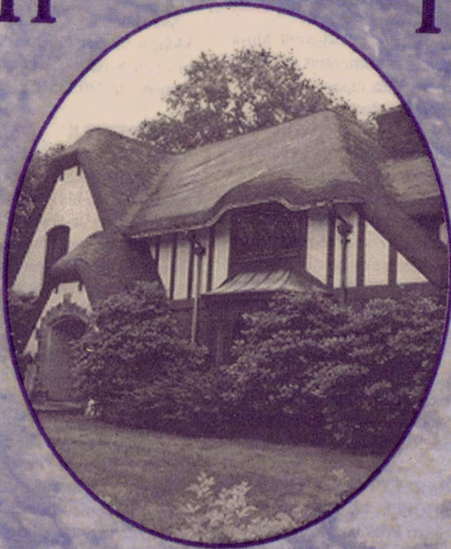
THE WAYNE A. YOUNG RESIDENCE, A COTSWORTH COTTAGE AT 221 BROAD STREET, WAS BUILT IN 1926. ROY FIRESTONE WAS THE ARCHITECT. THE YOUNG FAMILY TURNED THE HOME OVER TO THE METHODIST PARSONAGE IN 1959.
